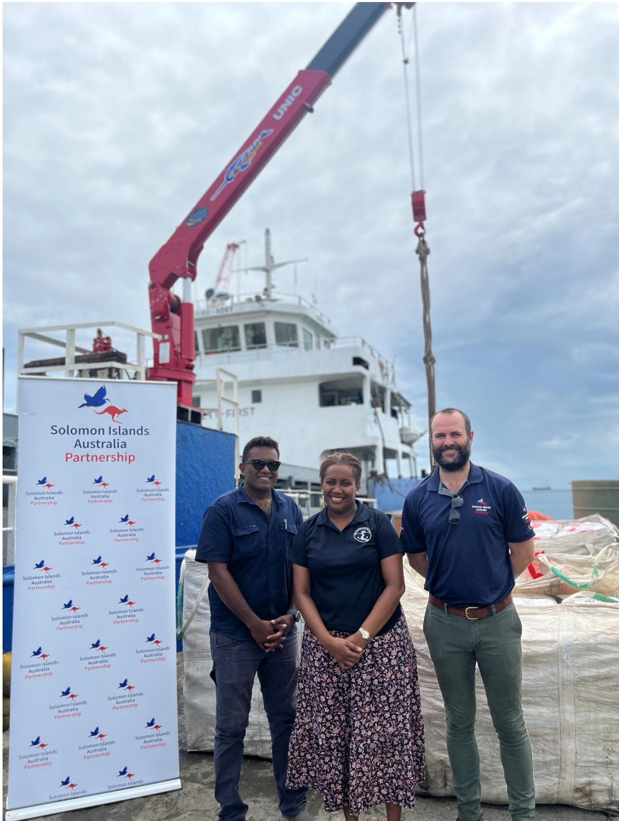
Caption 1: Australian High Commission First Secretary Economic, William Rowell, (right) with Joy Isihanua Ririmae and Alick Isihanua of Franjti Shipping Ltd standing in front of the newly installed crane on MV Florence. This is part of the Solomon Islands -Australia Partnership with Franjti Shipping Ltd to improve market access for cocoa and copra farmers in the Weather Coast of Makira through reliable shipping services.
